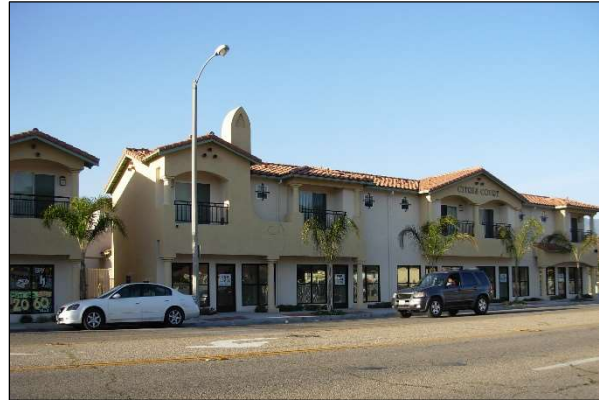
Citrus Court Apartments Mixed Use Project
